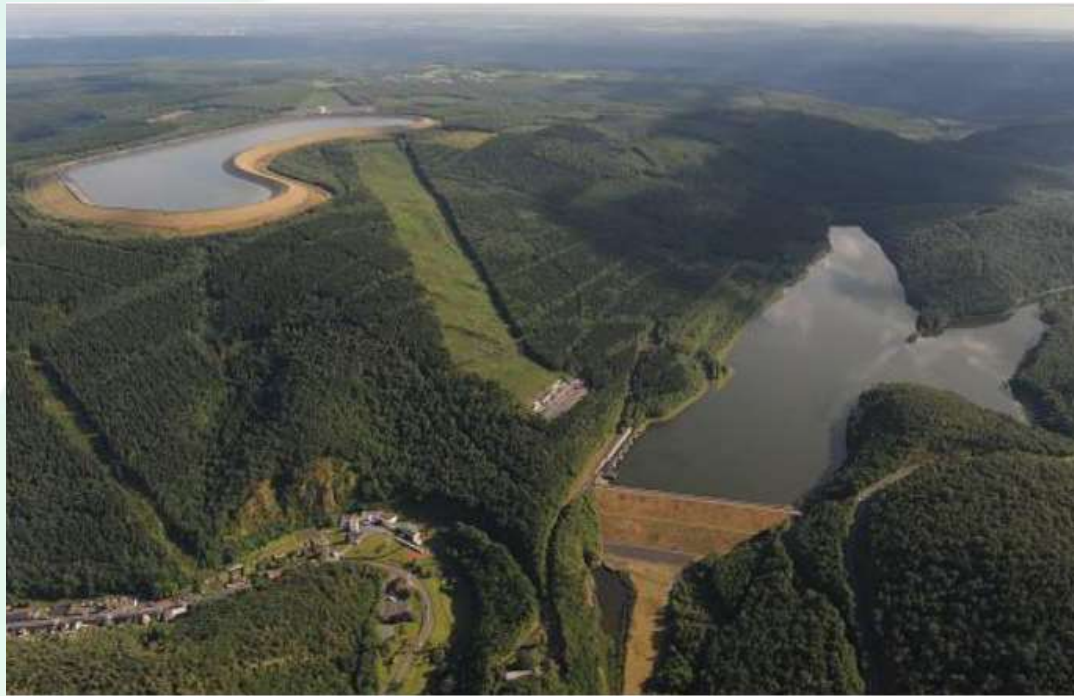
Pumped Storage Hydropower at Revin (Photo EDF)
